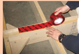
1 Installation on bond-breaking tape
