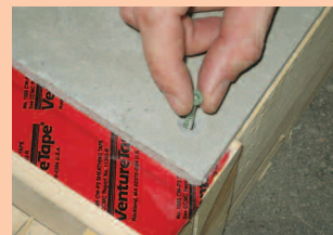
4 Hole must be larger than diameter of screw
